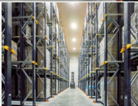
Can be used with either LIFO (Last in, First out) or FIFO (First in, First out) when there are more than three lanes per SKU.
