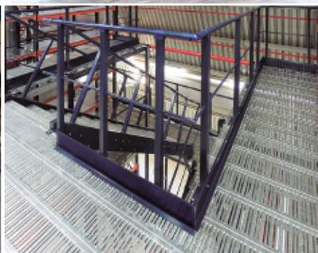
Mezzanine floors can be completely disassembled and reused.
