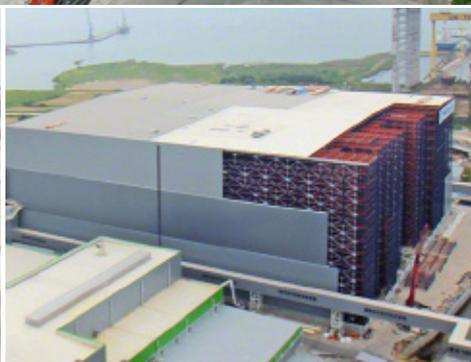
Clad-rack warehouses can use either automated systems or pallet racking, drive-in and cantilever racking, or the Pallet Shuttle, etc.
