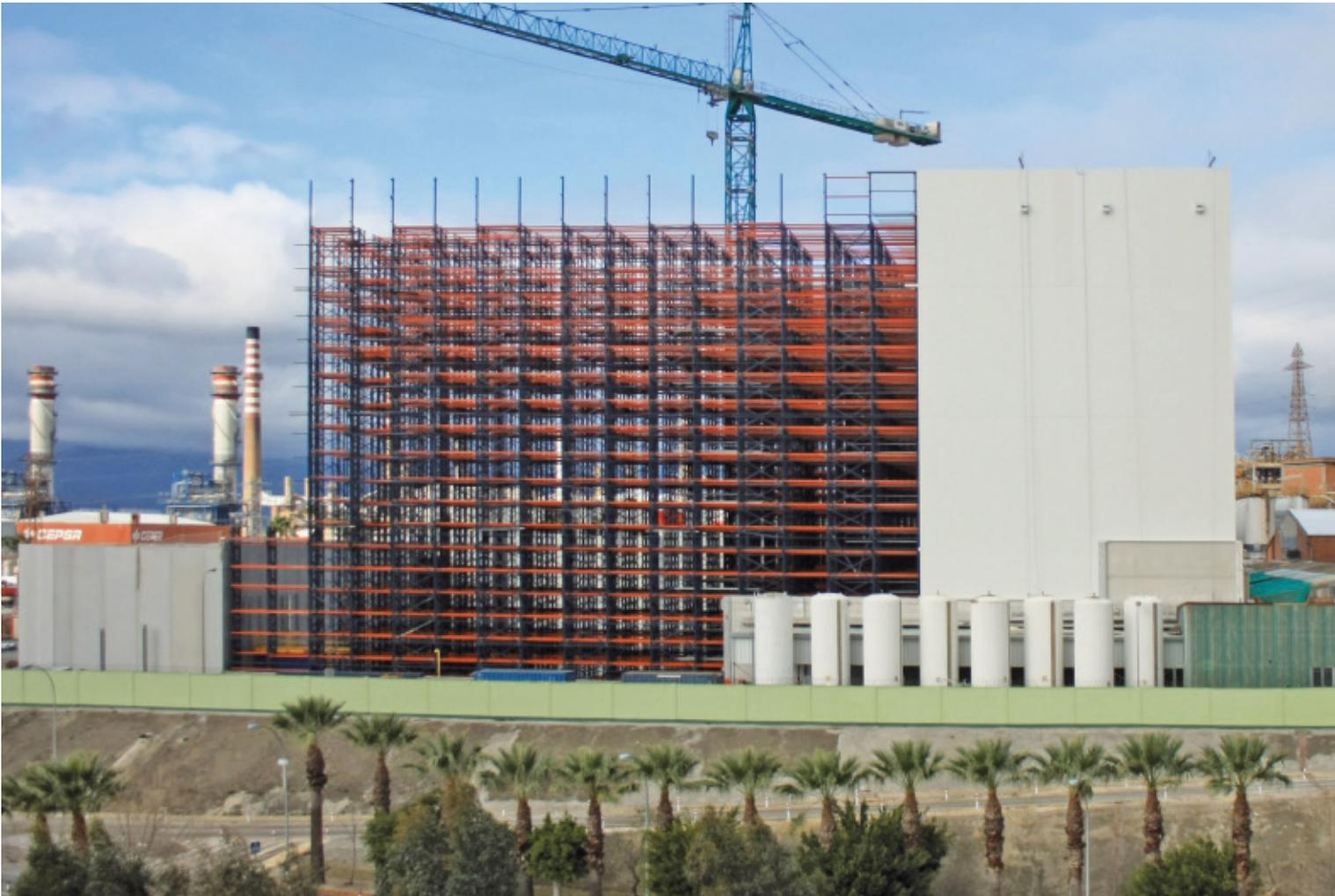
The clad-rack warehouse is the ideal solution for stacking goods high, as its design ensures the racking structure forms a compact unit along with the roofing and the cladded walls of the warehouse, removing the need for building work.
